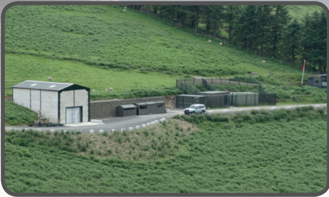
Indoor range and large workshop and target area.
